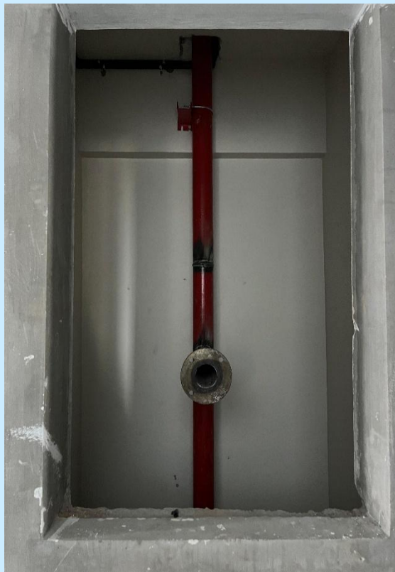
T1 FIRE RISER INSTALLATION
