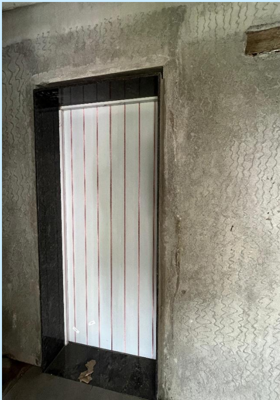
T1 LIFT JAMBS GRANITE FIXING
