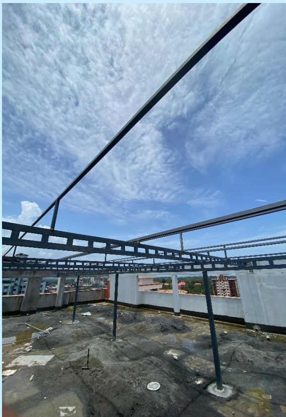
T2 ROOF TRUSS FOR SOLAR
