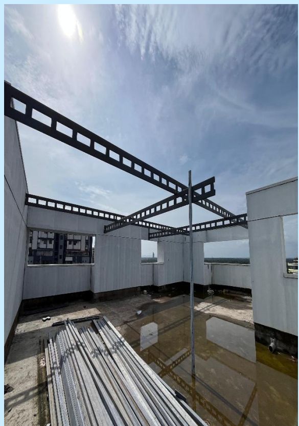
T1 ROOF TRUSS FOR SOLAR
