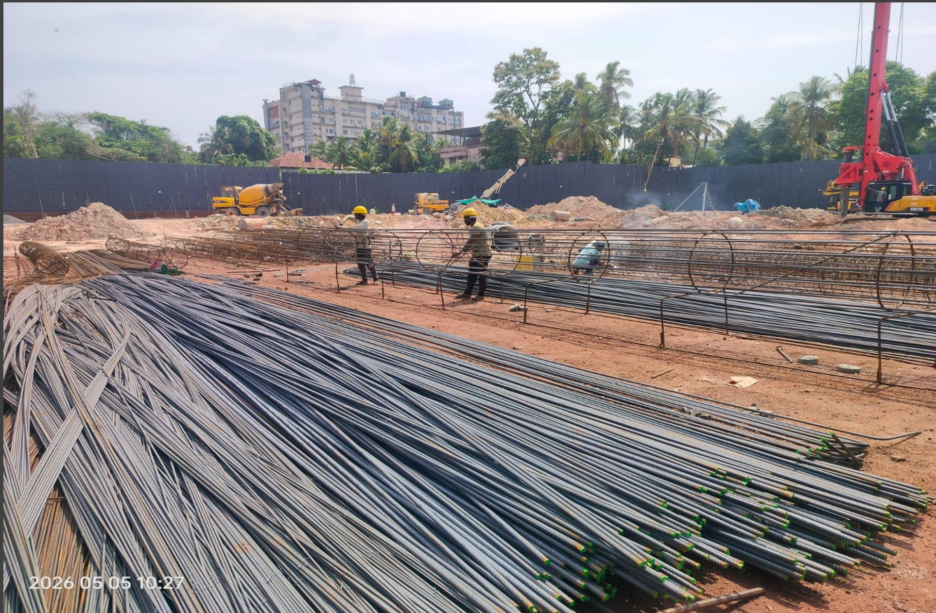
REINFORCEMENT CAGE FABRICATION
