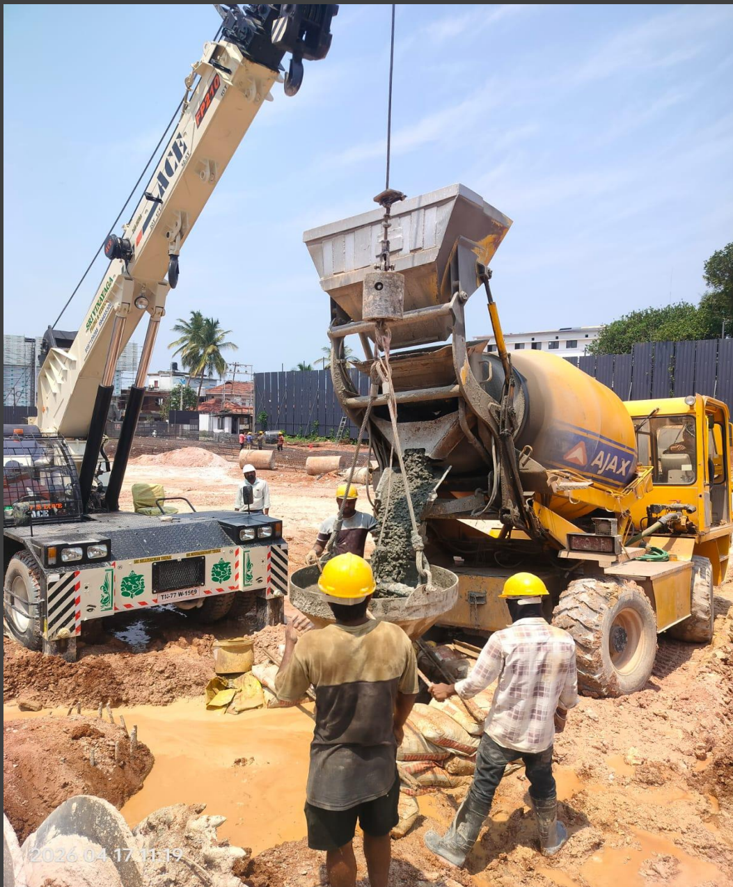
PILE CASTING
