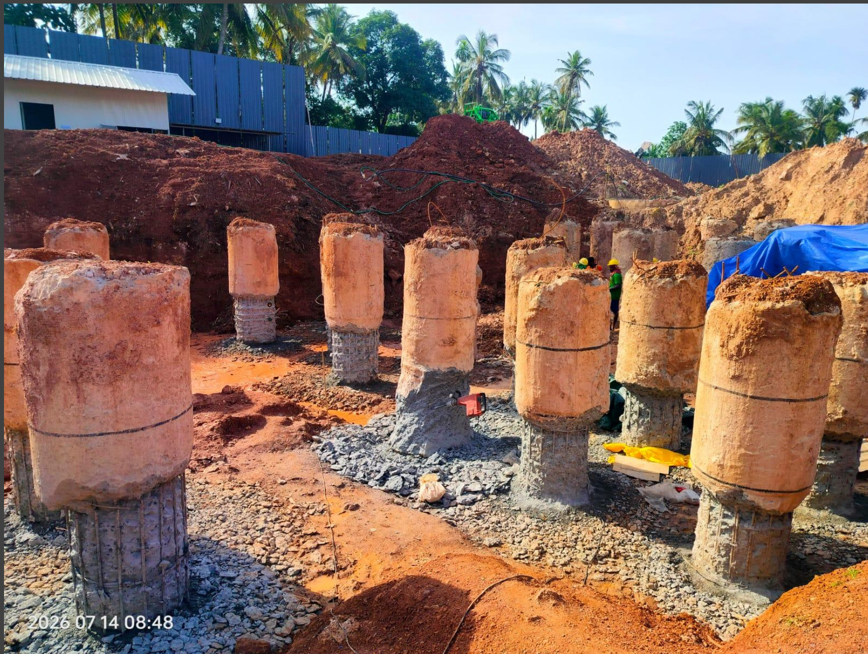
PILE CHIPPING WORK
