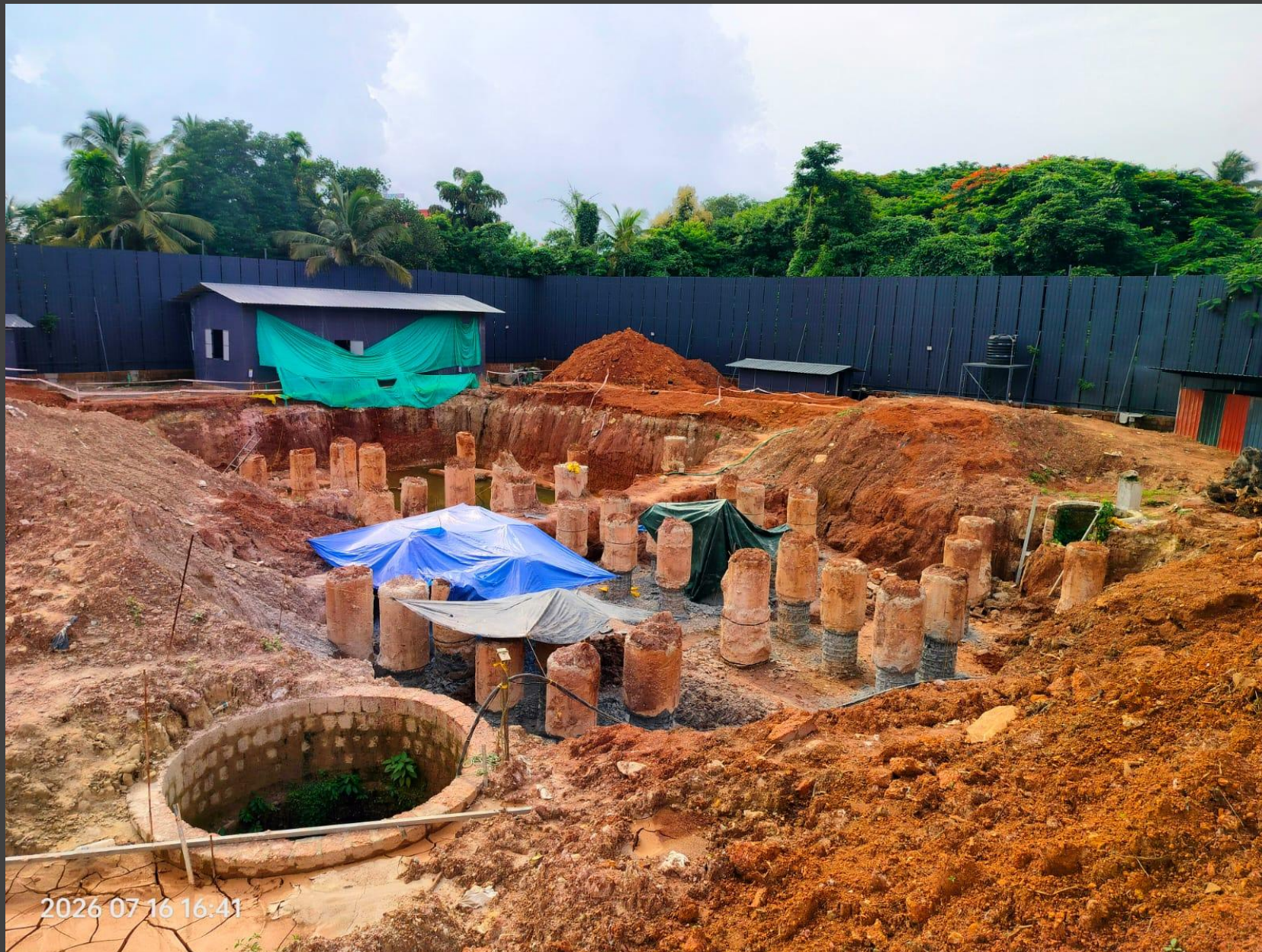
PILE CHIPPING WORK
